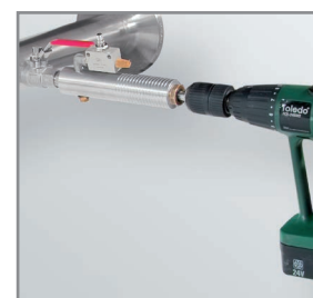
Drilling under pressure with CS drilling jig
