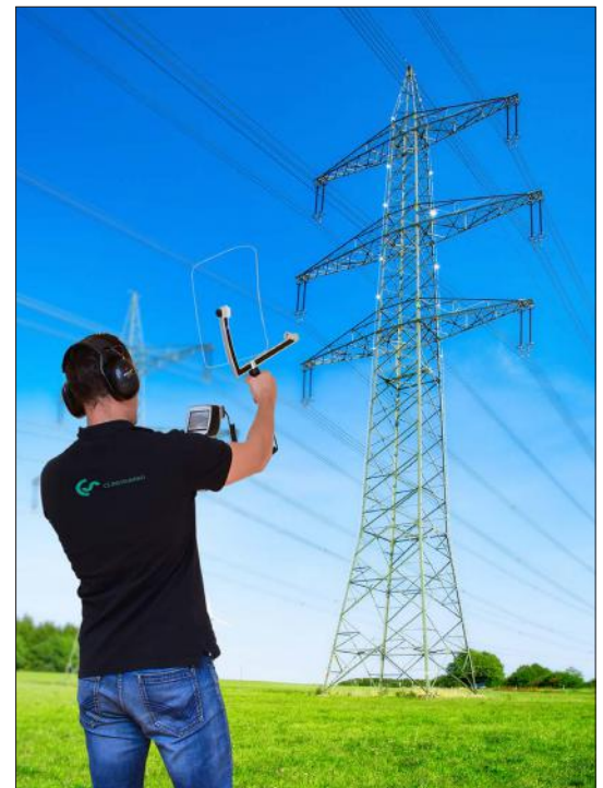
Checking high voltage overhead lines for corona discharge
